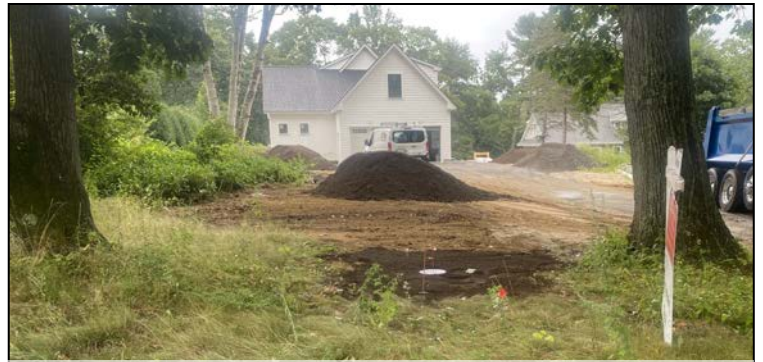
30 Southside Road one-inch plastic meter pit installation
