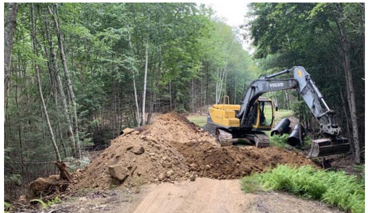
Digger's Excavating replacing a 24-inch culvert on the Red Management Road
